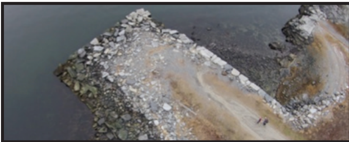
Aerial view of the Stone Dock prior to reconstruction.
